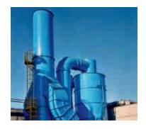
Our dry scrubber combines carefully chosen chemical reagents with exhaust stream at incredibly high speed that react with or absorb the compounds in the stream. The working diagram has been shown.
