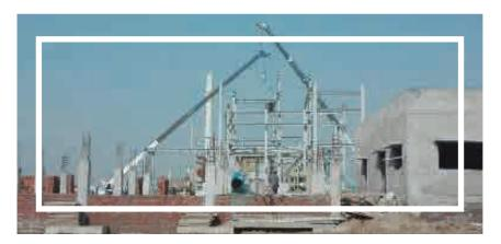
enables a wide range of radii to be achieved quickly and easily compared to conventional crawler cranes. And what's more, the boom can even be extended and retracted with a load on the hook.
