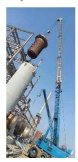
Crawler cranes with lattice booms move very heavy loads safely and economically. The telescopic crawler cranes are flexible in use and require very short set-up times. The telescopic boom whose concept has been adopted from all-terrain cranes.
