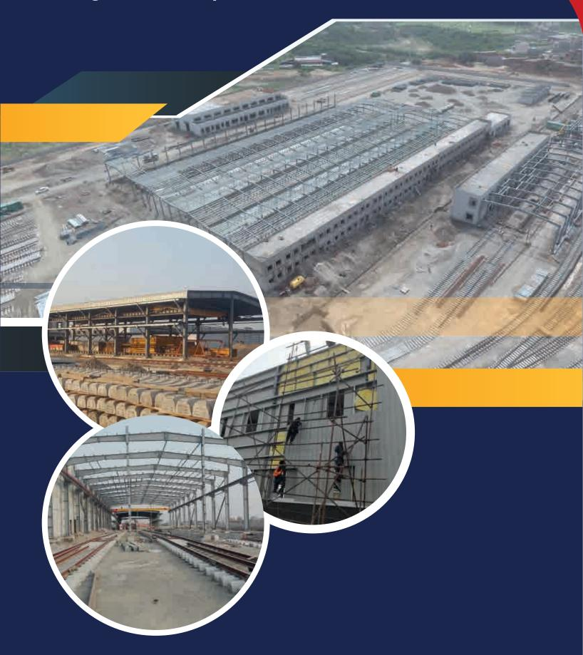
PRE-FABRICATED BUILDINGS OF COVERED AREA 56,500 m<sup>2</sup> FOR ORANGE LINE TRAIN DEPOT LOCATED AT DERAN GUJRAN, LAHORE
